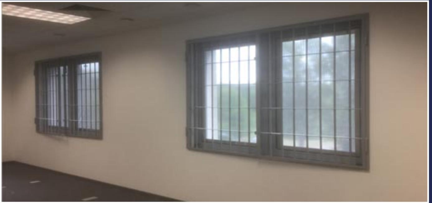
Electromagnetically shielded room, the picture shows windows with see-through electromagnetic shielding.
