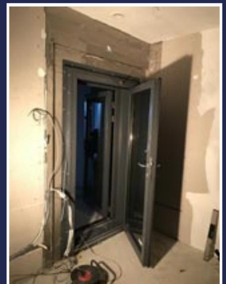
After the electromagnetic shielding is installed, a documented measurement of the electromagnetic attenuation is carried out separately for each building partition surrounding the secured room.
