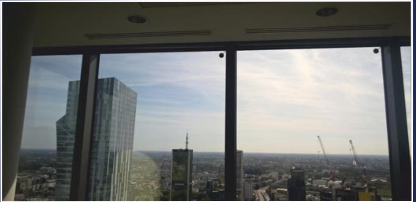
Vibroacoustic protection on the windows with PIEZO transducers visible in the upper right corners of window panes.
